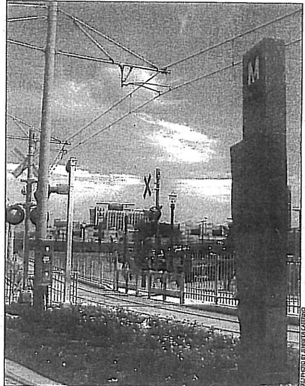
The first stop of Metro's Gold Line Eastside Expansion is being completed in Los Angeles' Little Tokyo/Arts District. Another proposed extension will continue the Gold Line from its current end in East Pasadena to Montclair. A final leg connecting the route to L.A./Ontario International Airport depends on funding and completion of the light rail's San Gabriel Valley extension.
