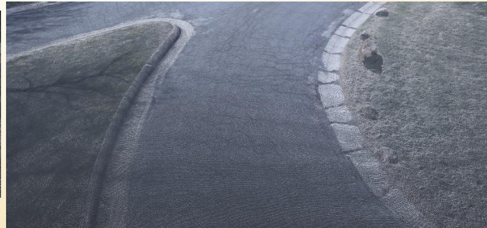
LIDAR Generated 3D Images showing Pavement Distresses for Ginger Bend
