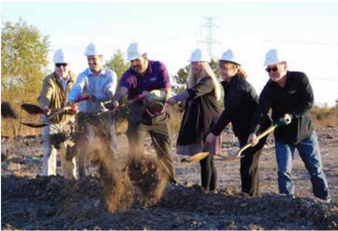
Donco Electrical Construction & Fowler Management Services, November 9
