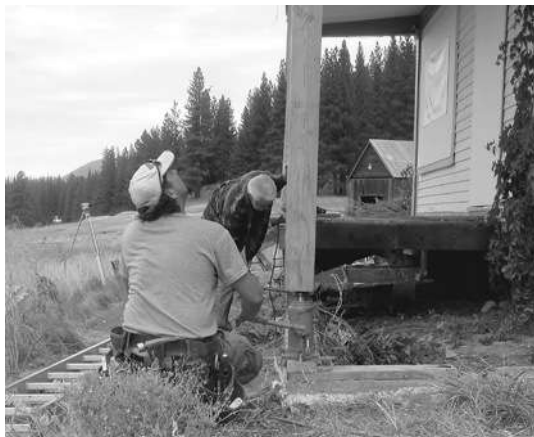
Erik Roosenschoon (foreground) and Jim Harper man the jacks to raise the sagging balcony at White Sulphur Springs Ranch.
