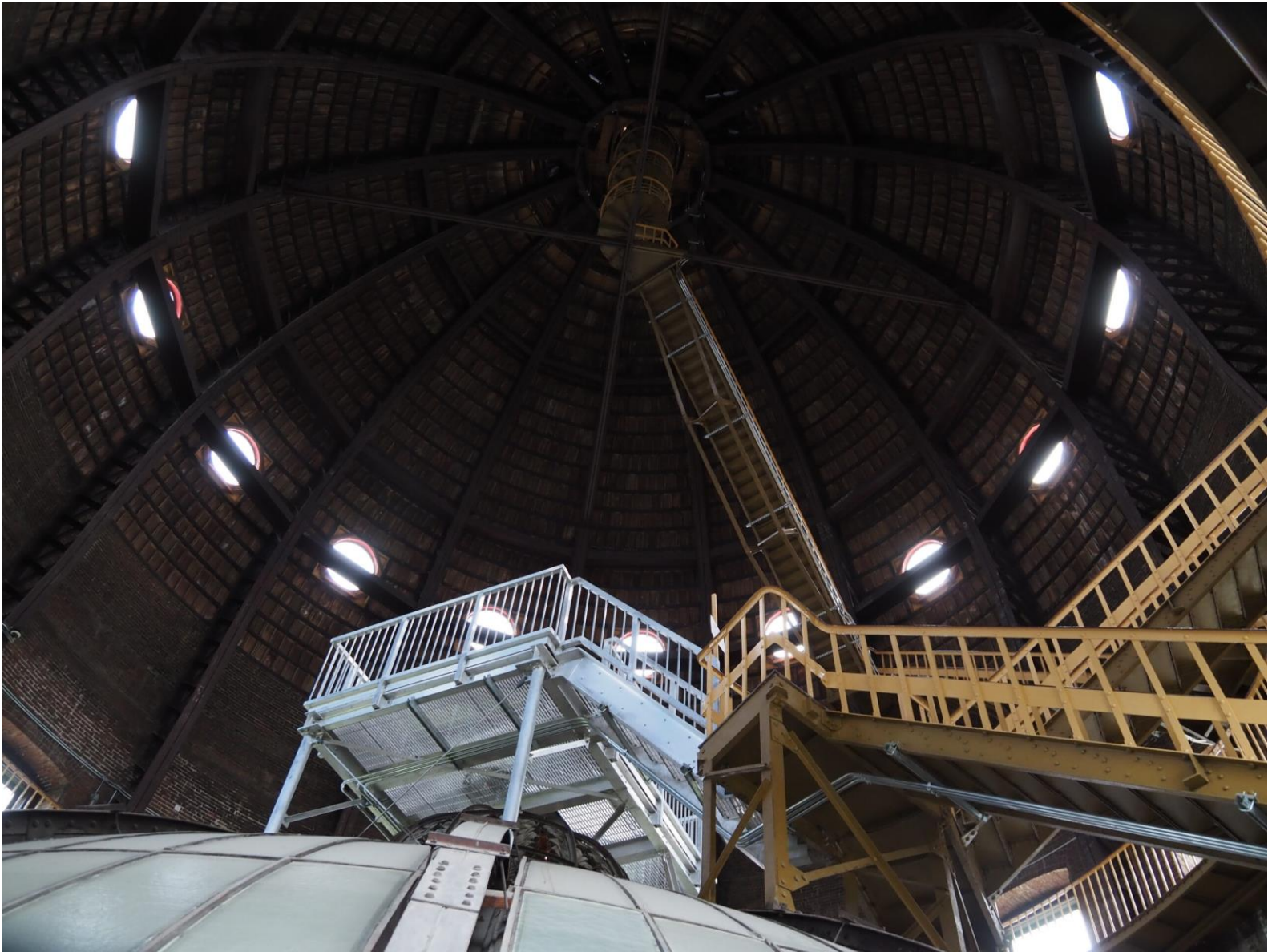
Looking up once above the inner dome
