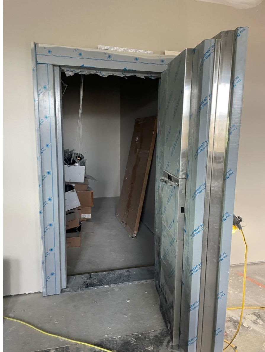
The new vault
