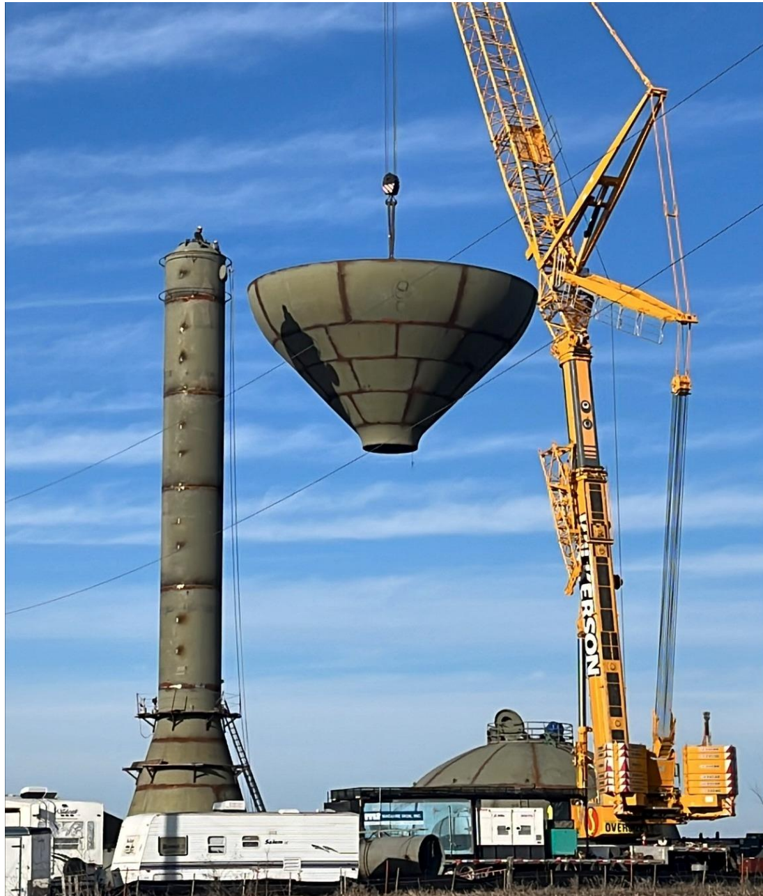
Piecing together the tower
