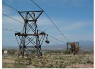
y This aerial tramway operated in the 1920's and 1930's carrying ore from the mines on Treasure Hill to Godbe's Mill in the valley. Built by Pioche Mines Company, the tramway was mainly gravity powered with the aid of a 5 horsepower motor. The ore in the full buckets rolled toward the mill and provided the momentum to return the empty buckets to the bin. In 1928 the cost of delivering ore to the mill via this tramway was six cents per ton.
