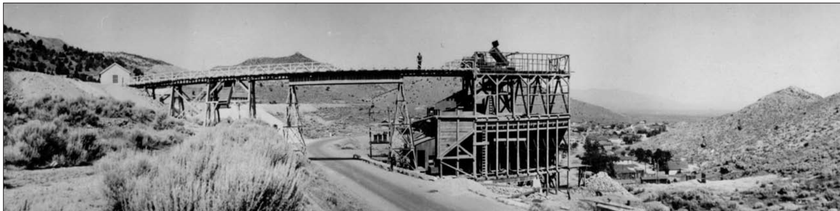
Trestle and ore bin for Pioche Tram.
