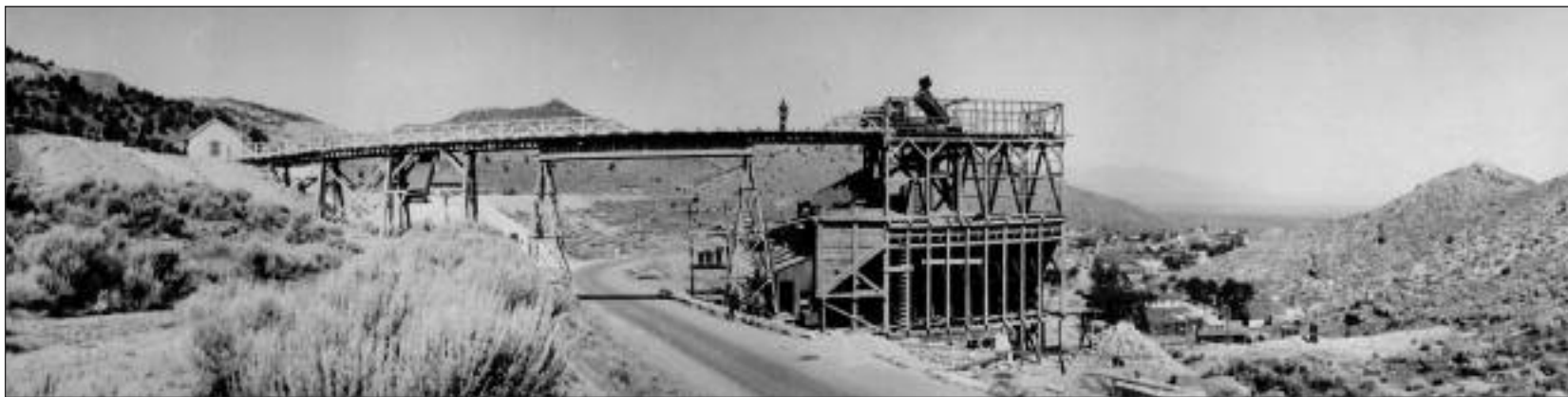
Trestle and ore bin for Pioche Tram.
