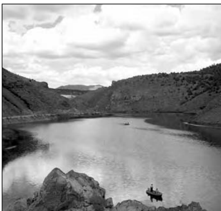
Eagle Valley Reservoir
